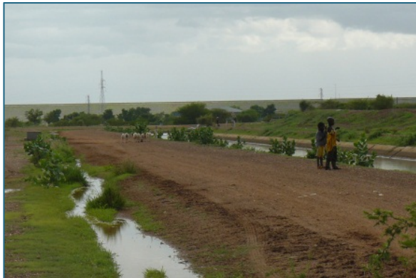
Bagré irrigation scheme
