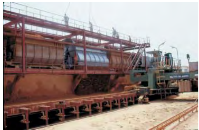
Figure Togo 7. Togo Beneficiation Plant, Ore Offloading Station
