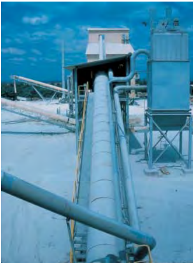
Figure Tanzania 7. Minjingu Beneficiation Plant, Initial Crushing Station
