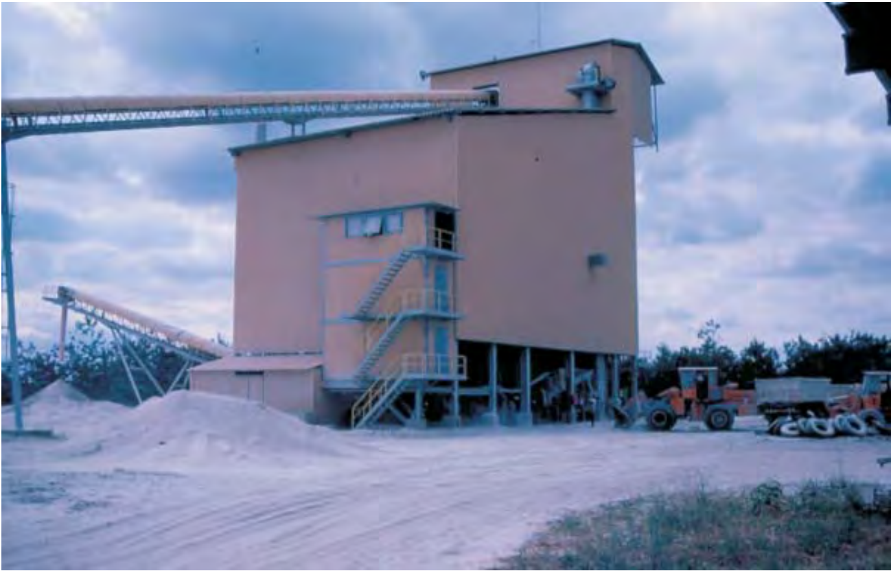
Figure Tanzania 8. Minjingu Mine, Main Beneficiation Plant
