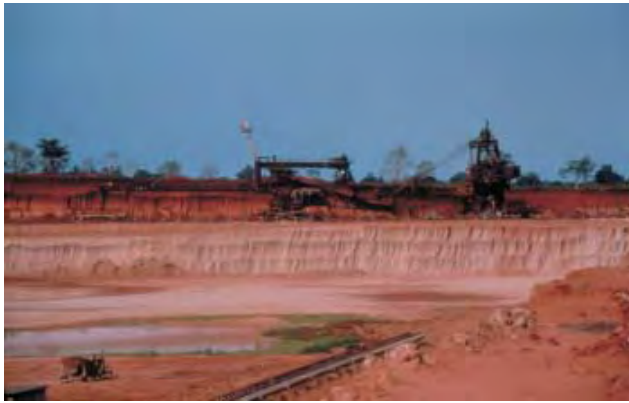
Figure Togo 4. Kpogame Mine, Togo, Overburden Stripping
