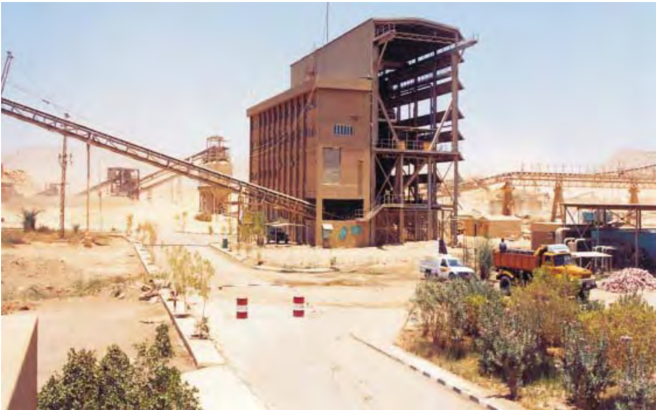
Figure Egypt 3. East Sebaiya Area, Washer Plant, ENMC Office Area
