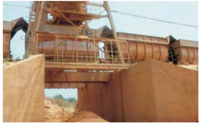
Figure Togo 6. Kpogame Mine, Rail Transfer Point
