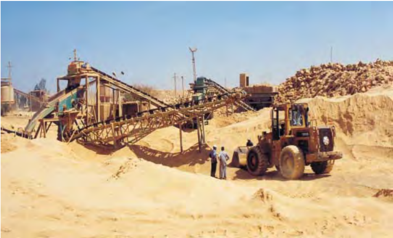
Figure Egypt 2. East Sebaiya Area, Small Crusher, ENMC Office Area
