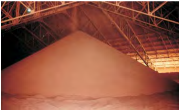
Figure Togo 13. Togo Beneficiation Plant, Storage Shed
